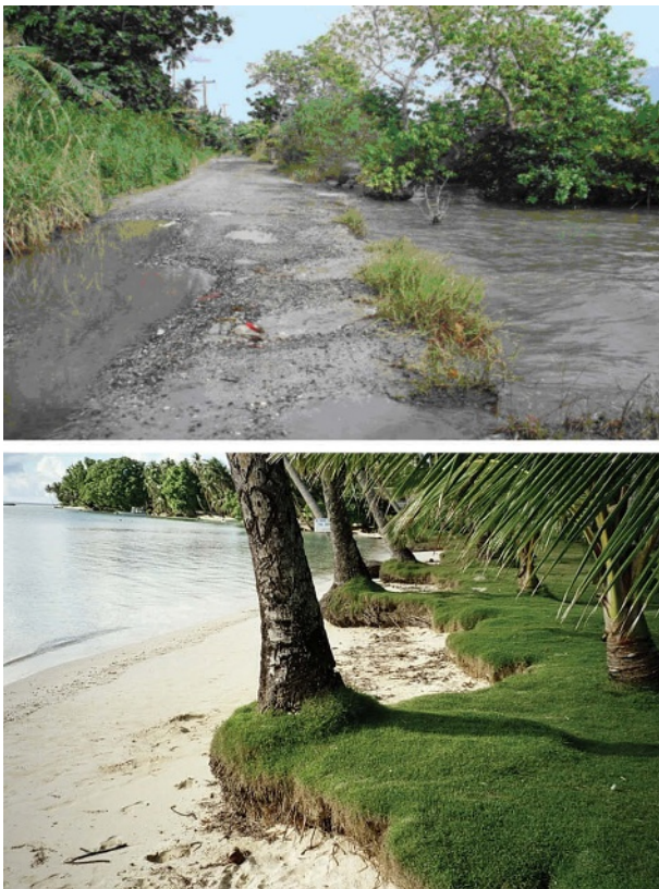
FIG. 6. (top) Inundated roads in Wichap Village (Weno, Chuuk, FSM); photo courtesy of J. Berdon, WSO Chuuk, and (bottom) results of coastal erosion at Blue Lagoon Resort (Weno, Chuuk, FSM) during the La Niña of 2007/08. [Photo courtesy of C. Guard, WFO Guam.]
